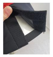
2. Unfold the fabric and open the velcro flap at the bottom. Fit the fabric around the duct, ensuring that the velcro strips on the bottom of the duct line up with the velcro strip on the bottom of the fabric. Finish installing the fabric by closing the fabric flap and lining up the velcro on either side of the flap.
